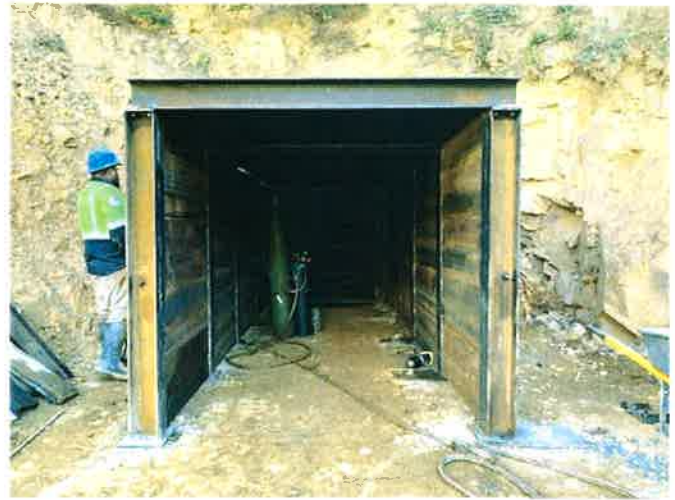
Portal Repair Work at Yukon Mine
