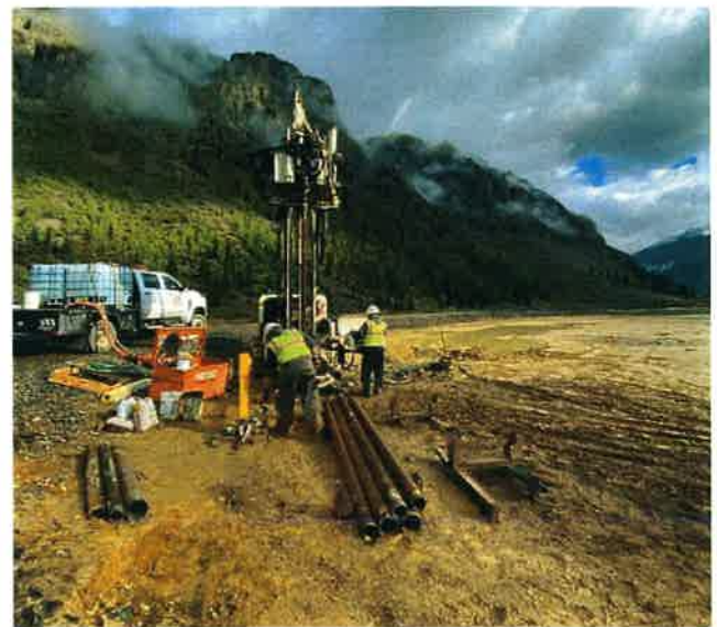
Well Installation at Howardsville.
