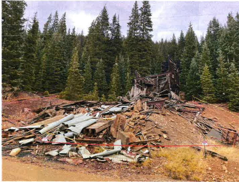
Figure 1. Overview of Lead Carbonate mill structure slated for demolition. Junk with no historical significance in foreground, dilapidated middle structure probably not worth saving, intact ore bin at far end.
