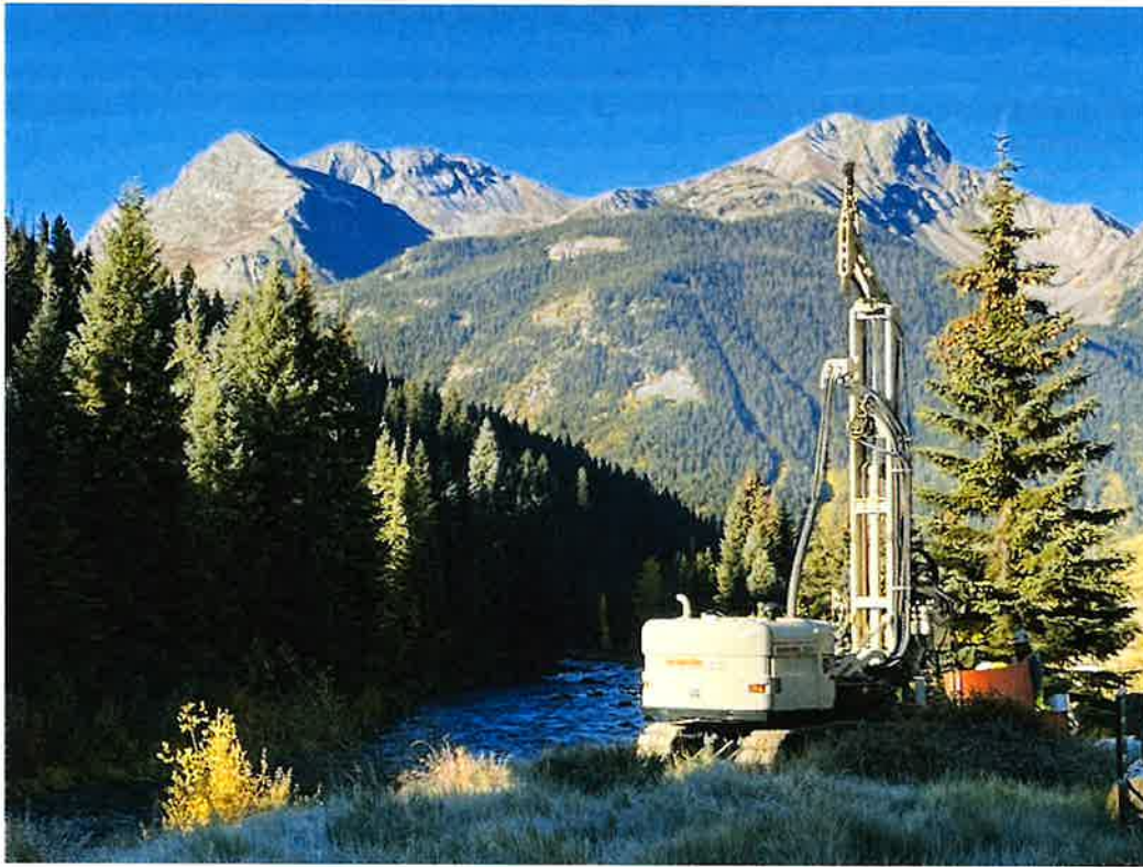
Monitoring well installation at the BPMD Site – Photo taken on September 25, 2025
