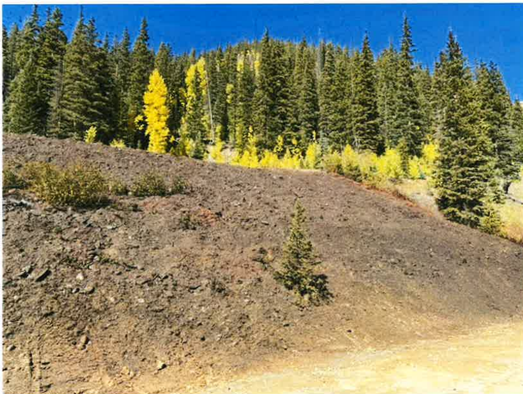
Stabilized hillside where old crib wall was located – Photo taken on September 24, 2025
