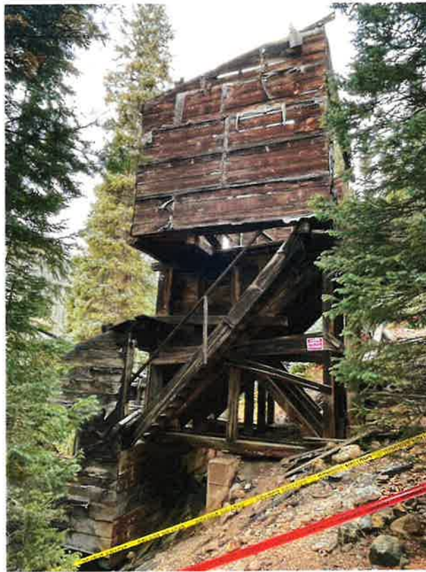
Figure 3. Lead Carbonate ore bin in relatively good condition and worth saving from demolition. View to north of south side.
