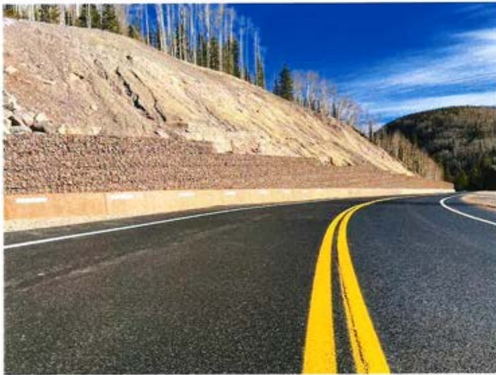
Completed slope work and rockfall catchment barrier on US 550 at the Deer Creek location (MP 59.3)
