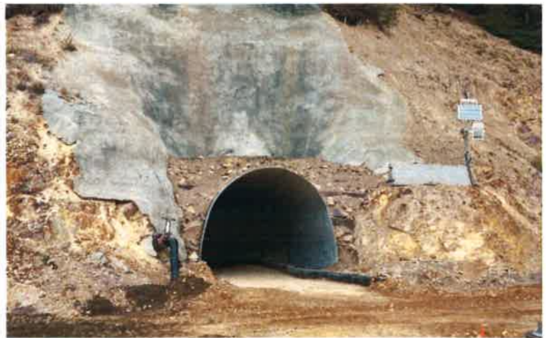
Completed portal extension at Gold King Mine
