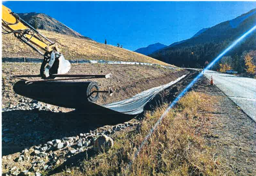
Stormwater channel along County Road 2 being lined prior to backfill
