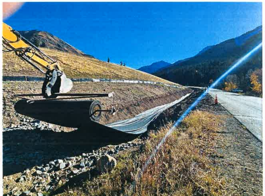
Liner installation in a stormwater channel of the Bonita Peak Repository
