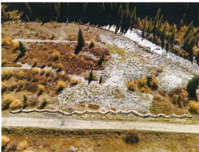
Aerial view of fencing installed at Campground 4
