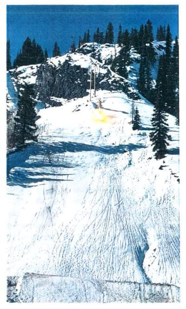
Permanently installed avalanche mitigation equipment uses compressed area and gasses to trigger slides on US 550 Red Mountain Pass.
