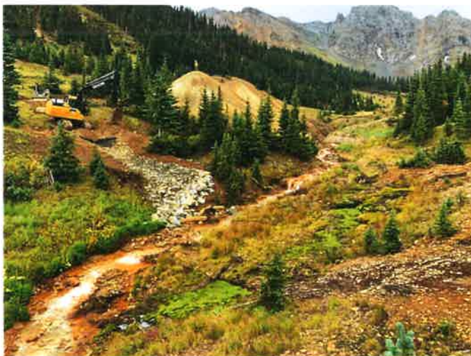
Figure 3 Before IROD work (left) and channel being created to divert adit discharge around waste pile (right)
