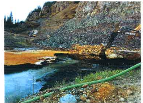
Figure 2: Kohler Tunnel sediment removal
