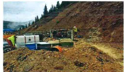
Figure 2: Gold King Mine borehole work
