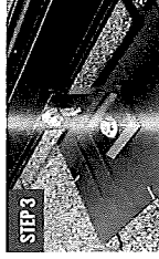
ATTACH L-FOOT TO RAIL
