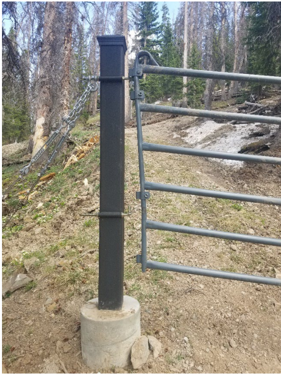
Gate damaged by snow creep Survey pin in post foundation
