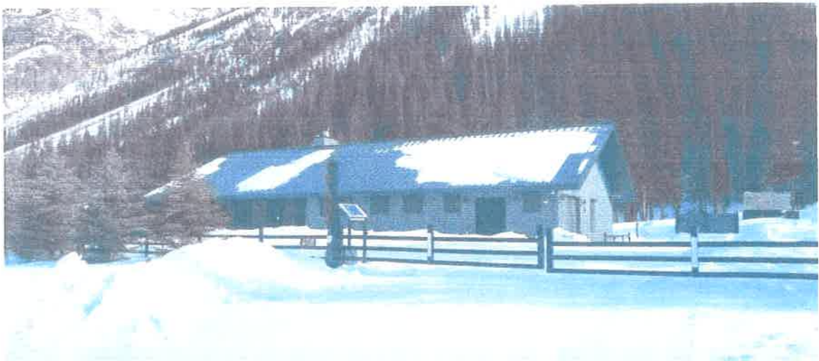
Photo taken from County Road 2 facing east towards the new existing Riley residence, and existing fence/gate. The style of the proposed fence extension will match the existing matte-black-painted metal fence shown in the picture.
