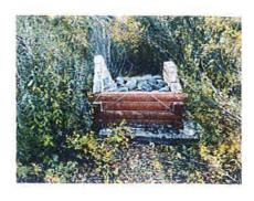
shown in the above righthand picture are holding down wooden boards sealing off critter access to the well.
