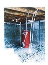
inch T&G ply-board to support future snow loads. It would also need something such as an epoxy coating as weather protection. The total abovegrade height would be about 16 inches, a height that survived the previous avalanche. The goal is to create a secure, protected area for stored personal property and water well hardware and plumbing. Pictured is the undamaged pressure tank for the water
