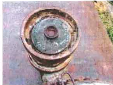
Breather (vent) valve close-up. Cast iron, made by "M. L. Hayden Mfg. Co. – Columbus, Ohio"
