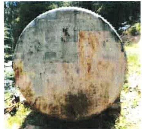
Flat tank end
