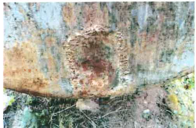
Bottom end view (perhaps an old drain?)
