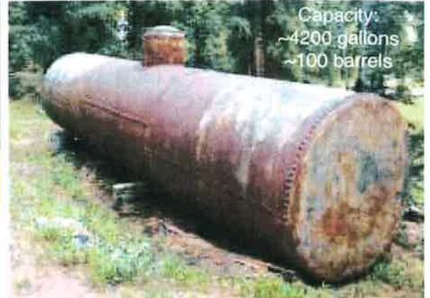
Tank side and quarter views – 24-ft long, 5-ft 7-in. diameter. Three courses of 0.25-in. steel plate; pointed rivets 2-in. apart. Welds and marks for old hand grabs, hand rails, and straps.
