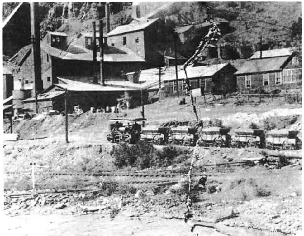
Vanadium Mill with Primos Chemical Company improvements. Note the crawler tractor pulling wagons of ore. It replace a team of mules.
