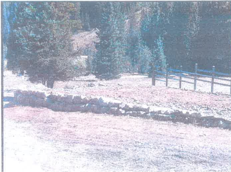
Photo provided by the Applicant, showing the end of the existing fence, and the new existing septic area on Lot 2, as viewed from alongside County Road 2, looking towards the east-northeast.
