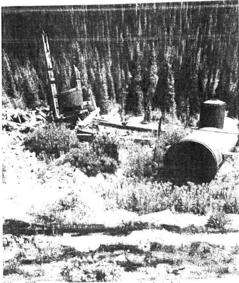
Boiler and machinery on the site today
