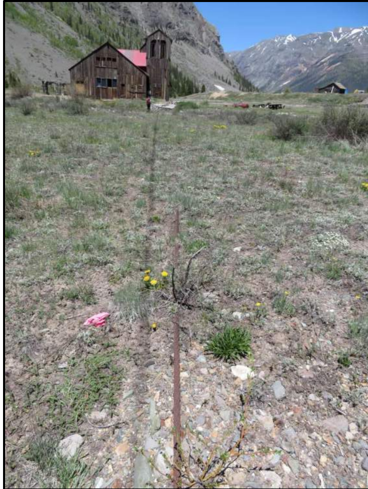
Figure 13. Little Nation Tramway line on ground and above leading to Little Nation Mill in the distance, looking north-northeast.
