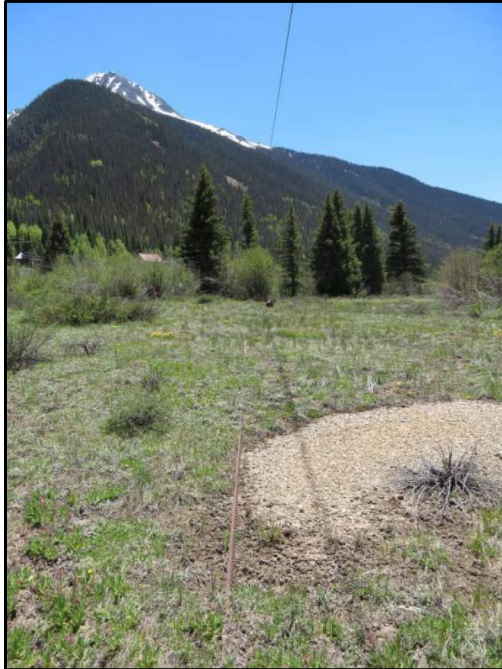
Figure 14. Little Nation Tramway line laying on ground and visible above leading to the Royal Charter Mine on the slope of King Solomon Mountain. View is to the south-southwest.
