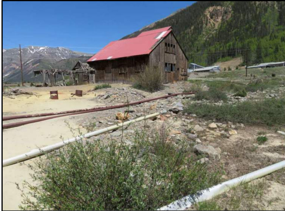
Figure 5. Little Nation Mill just north of the Winnemucca Mill Site showing aluminum and iron mill tailings slurry pipes passing over the northern portion of the Winnemucca Mill Site parcel. View is to the east-northeast.
