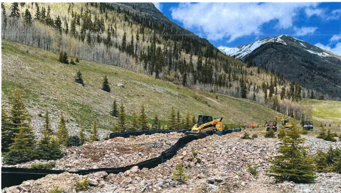
Repository construction on Tailings Impoundment 4 Photo: EPA
