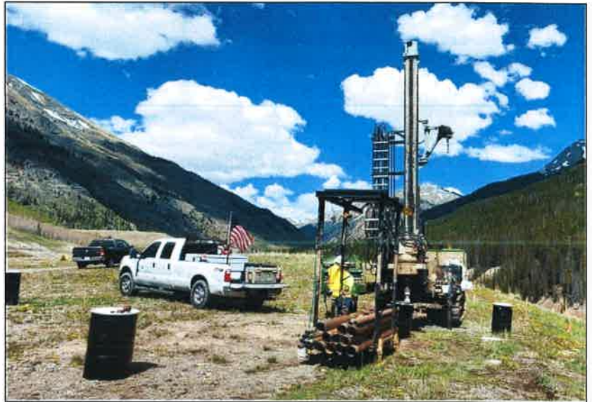
Preparations at the BPR: Drillers installing stability monitoring system
