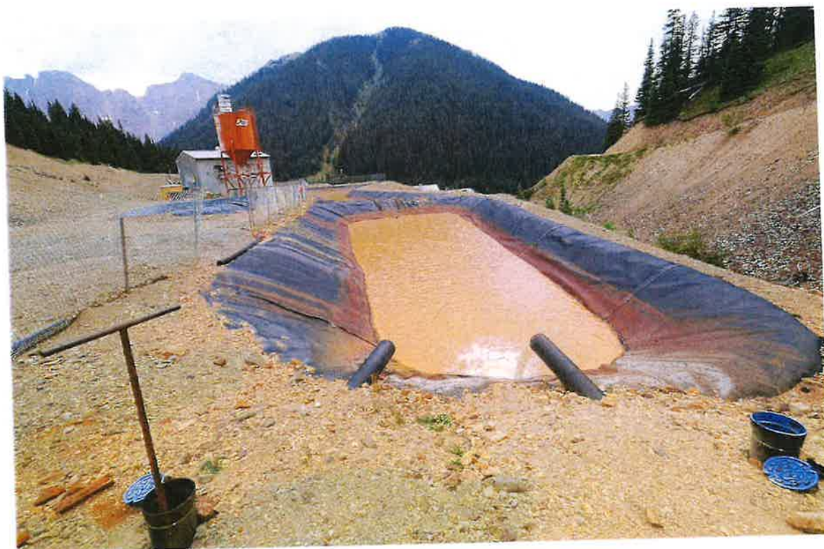
Water from the Gold King Mine flows into settling ponds on Wednesday before entering the Gold King treatment plant, which is about 3 miles north of Silverton. (Jerry McBride/Durango Herald)
