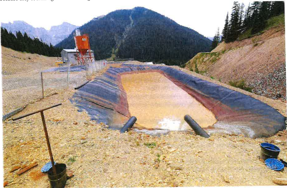
Water from the Gold King Mine flows into settling ponds on Wednesday before entering the Gold King treatment plant that is about 3 miles north of Silverton. (Jerry McBride/Durango Herald)
