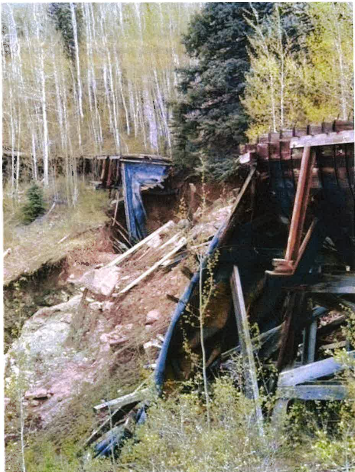
A flume collapsed near Cascade Creek in early June, causing terrain damage and threatening power line structures. (Courtesy of San Juan National Forest Facebook page, June 13).
