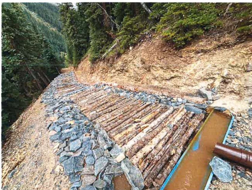
Iron terrace at Wynona Mine
