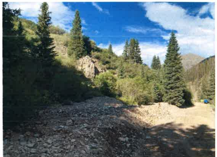
Clean fill material at trespass campground in July
