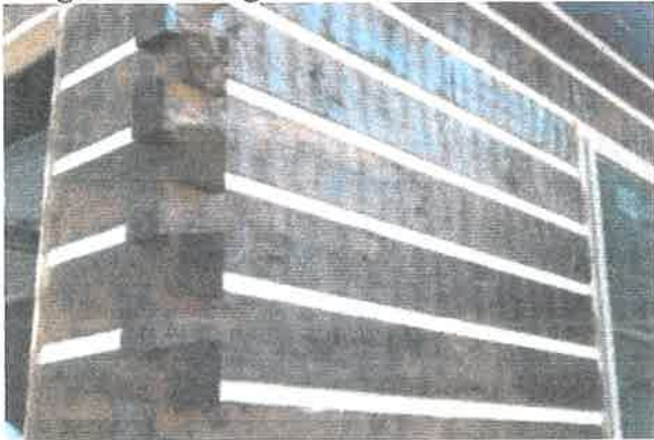
Example of Squared log cabin siding with white chinking. Image Credit: logcabinsforless.com
