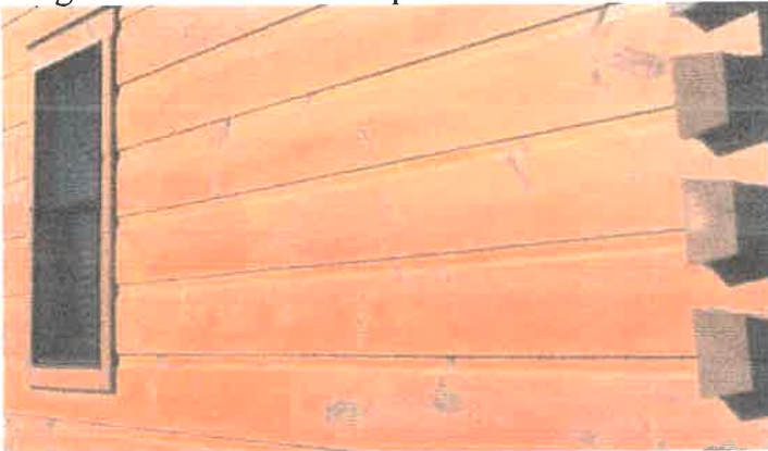
Example of Squared log cabin siding. Image Credit: Log Houses of America, Inc.
