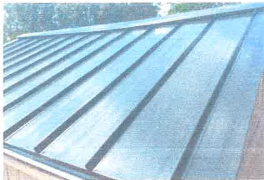
Dark or black standing seam non-reflective metal roofing (photo credit angleslist.com)
