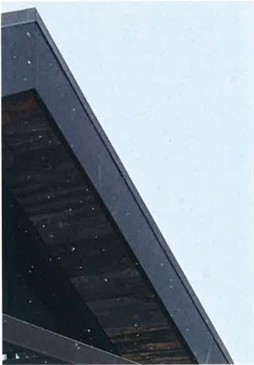
Faux barnwood soffit
