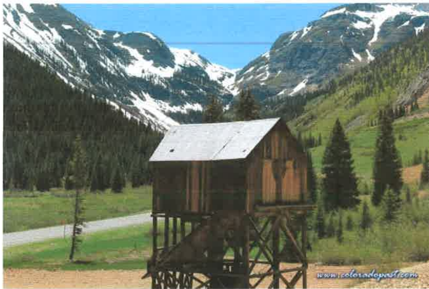
Silver Ledge Load Out Building
