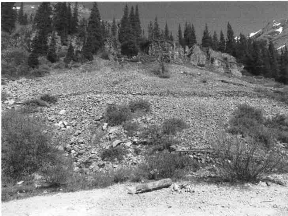
5SA407. View of the A-shaped avalanche deflector walls on the rocky slope west of the mine. View is to the west. Photo by Jon Horn, 6/20/2023.
