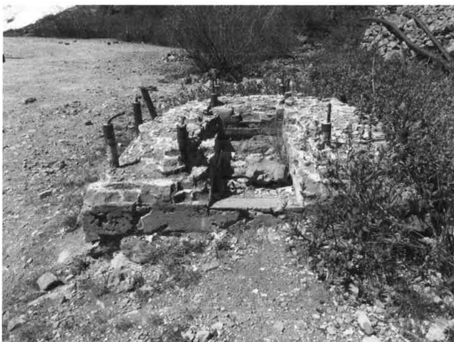
5SA407. Stone, cement, and brick compressor mount, looking south-southwest. Photo by Jon Horn, 6/20/2023.
