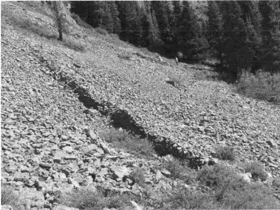
5SA407. A-shaped avalanche deflector walls looking north-northeast from the southern avalanche deflector wall. Photo by Jon Horn, 6/20/2023.
