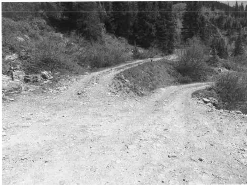
5SA407. Road switchback that has removed the boarding house/office and pushed it and artifacts downslope. View is to the north. Photo by Jon Horn, 6/20/2023.
