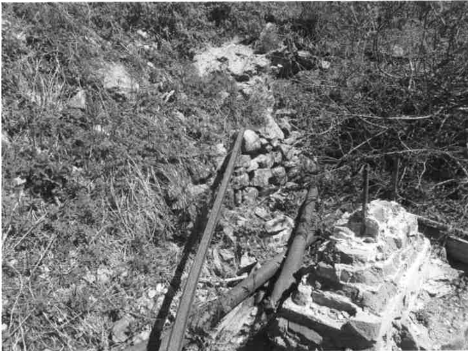
5SA407. Northernmost stone retaining wall remnant behind probable electric motor mount. View is to the north. Photo by Jon Horn, 6/20/2023.
