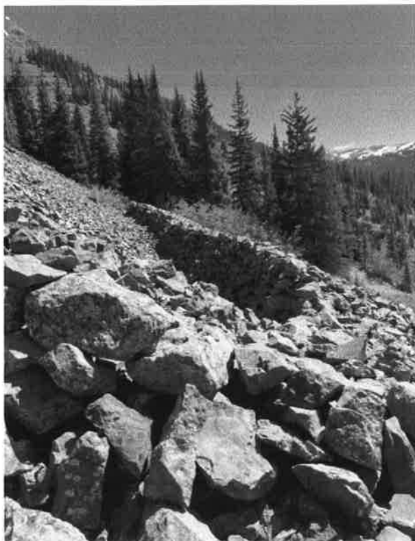
5SA407. The crossing wall of the A-shaped avalanche deflector, looking northeast. Photo by Heather Prosser, 6/20/2023.
