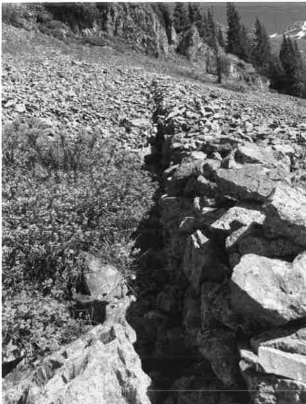
5SA407. Looking north-northwest along the western leg of the A-shaped avalanche deflector. Photo by Heather Prosser, 6/20/2023.
