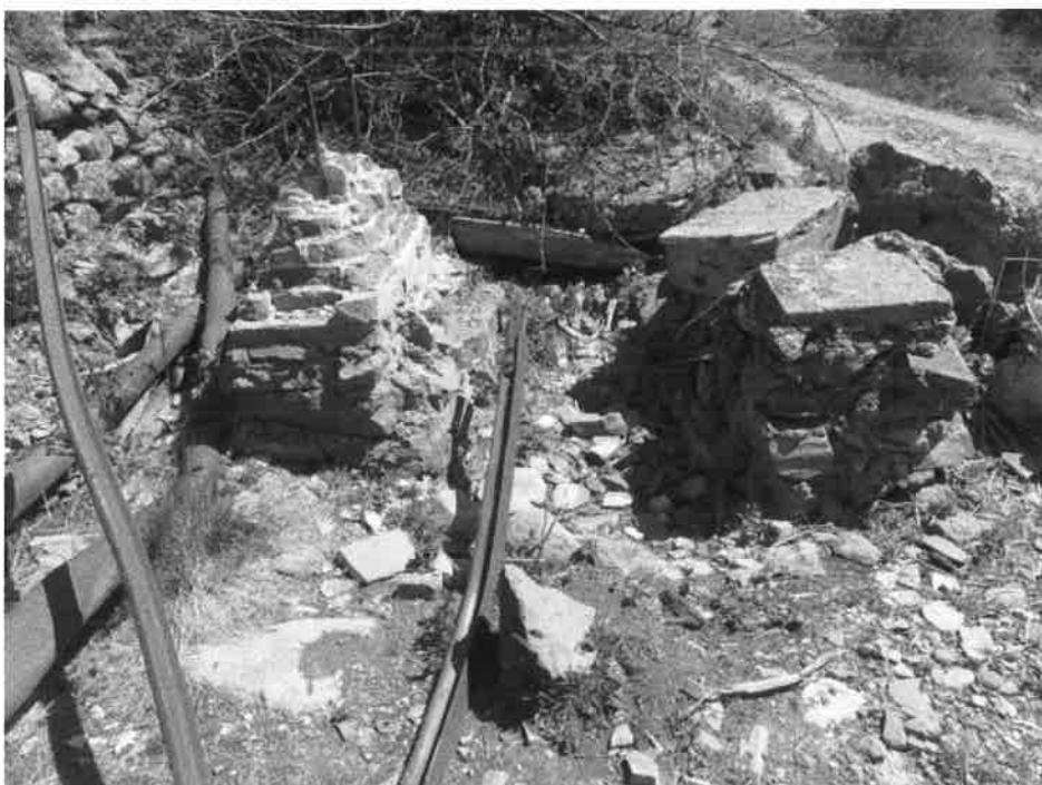
5SA407. Looking north-northeast at the probable electric motor mount with the building floor remnant behind. Photo by Jon Horn, 6/20/2023.
