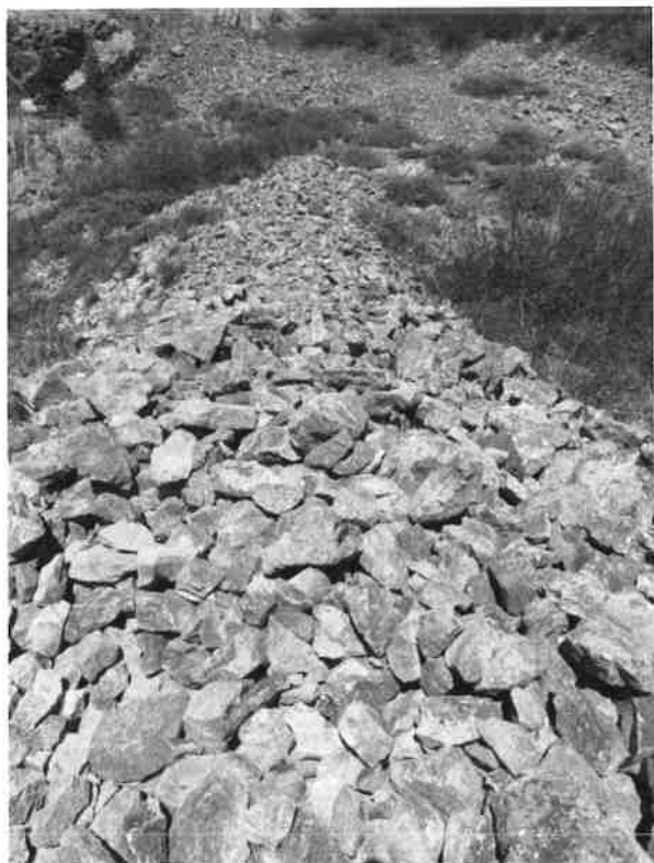
5SA407. Looking west along the southern avalanche deflector wall. Photo by Jon Horn, 6/20/2023.
