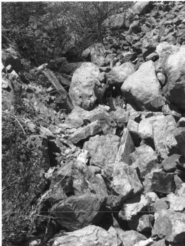
5SA407. Looking west at the collapsed adit with post and plank framing debris. Photo by Jon Horn, 6/20/2023.
