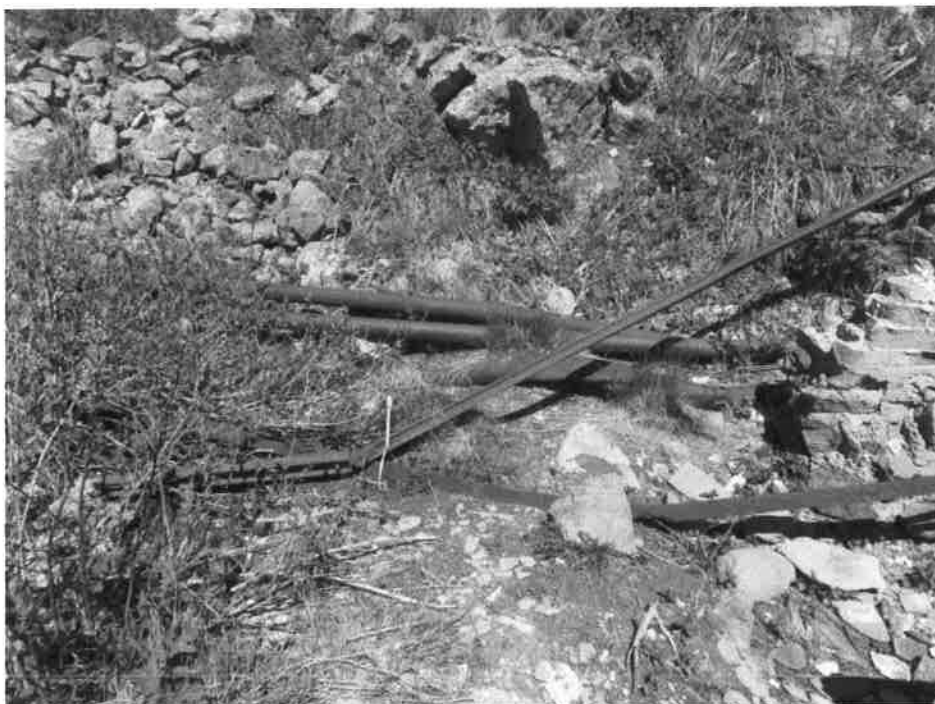
5SA407. Looking northwest at 4-in.-diameter iron compressed air pipe and ore car rail adjacent to the compressor mount. Photo by Jon Horn, 6/20/2023.
