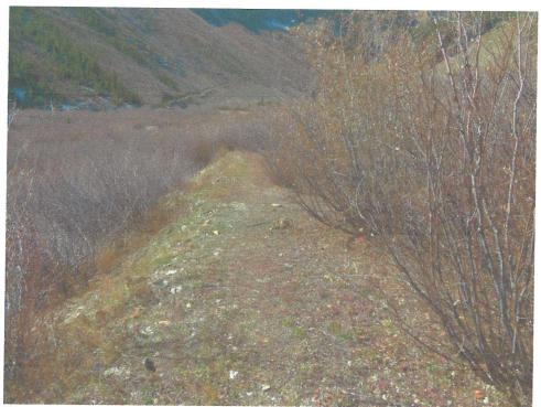
Figure 15. The main line grade (5SA112.16) partly covered with willows, looking southwest. Note the fill of the grade extending downslope to the left.
