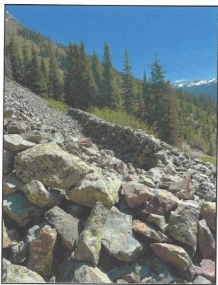
Figure 46. The crossing wall of the A-shaped avalanche deflector at the Silver Crown Mine (5SA407), looking northeast.
