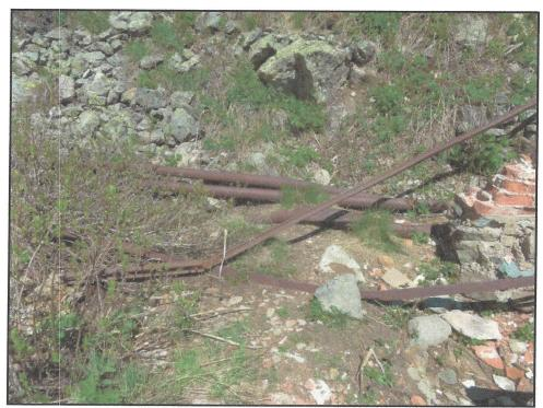
Figure 37. Looking northwest at 4-in.-diameter iron compressed air pipe and ore car rail adjacent to the compressor mount at the Silver Crown Mine (5SA407).
