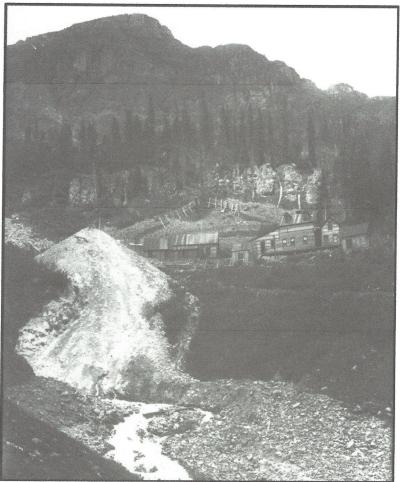
Figure 3. Silver Crown Mine showing the buildings constructed in 1906 with the avalanche splitting berms on the slope above.
