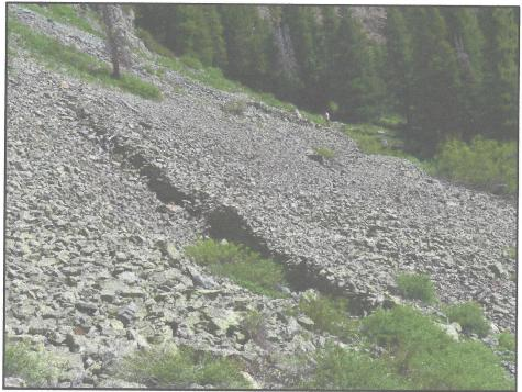
Figure 29. A-shaped avalanche deflector walls looking north-northeast from the southern avalanche deflector wall.
