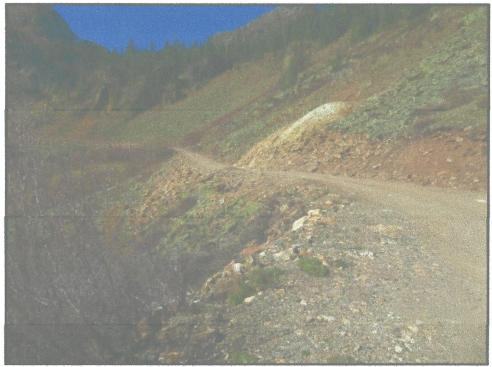
Figure 64. Cut and fill construction of Forest Serivce Road 821 (5SA1876.1) with the waste rock of site 5SA1875 visible near the center extending to the road. View is to the west.
