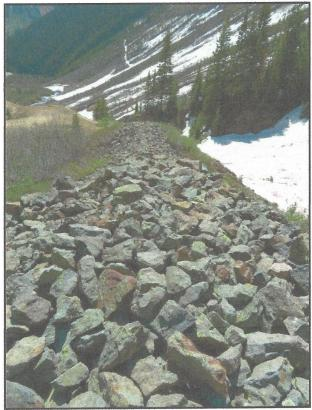
Figure 42. Downslope view of the southern avalanche deflector wall at the Silver Crown Mine (5SA407), looking east-southeast.
