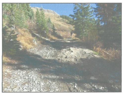
Figure 70. Forest Service Road 821 (5SA1876.1) above the Silver Crown Mine (5SA407) at the end of the recorded segment. Note the rough, eroded condition of the road with a slightly narrower width. View is to the east-northeast.
