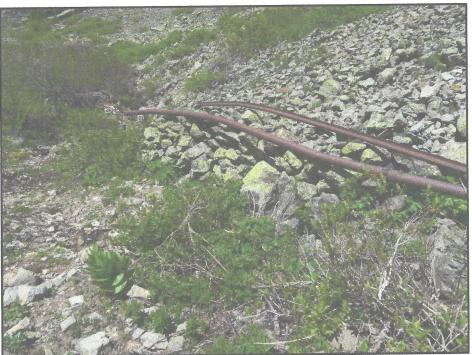
Figure 16. Looking west at the central retaining wall remnant with ore car rail and compressed air pipe disposed on it.
