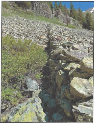
Figure 45. Looking north-northwest along the western leg of the A-shaped avalanche deflector at the Silver Crown Mine (5SA407).
