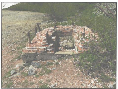
Figure 19. Stone, cement, and brick compressor mount, looking south-southwest.
