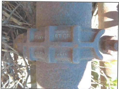
Figure 38. Victaulic pipe coupler on 4-in.-diameter iron compressed air pipe at the Silver Crown Mine (5SA407).
