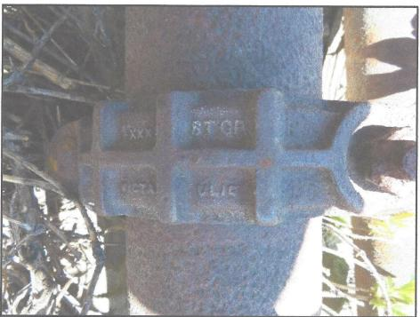
Figure 23. Victaulic pipe coupler on 4-in.-diameter iron compressed air pipe.
