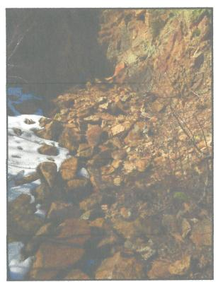
Figure 49. Mine adit of 5SA468 closed by filling with large angular cobbles and soil. Note the pipe with a brass cap on the end marking closure of opening No. 10 near the top of the cobble fill. View is up the adit trench to the west.
