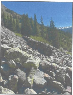
Figure 31. The crossing wall of the A-shaped avalanche deflector, looking northeast.
