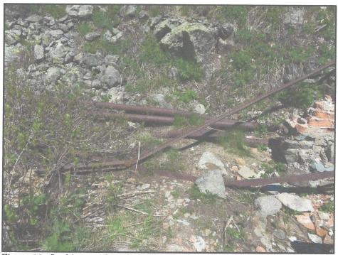
Figure 22. Looking northwest at 4-in.-diameter iron compressed air pipe and ore car rail adjacent to the compressor mount.
