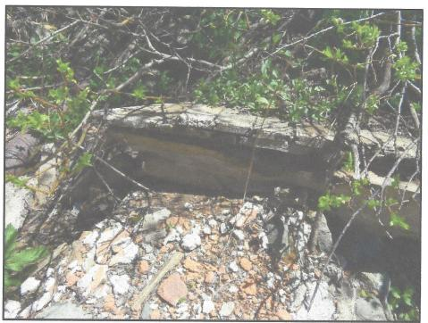
Figure 21. Building floor remnant showing diagonal 1-x-6-in. subfloor topped by 1-x 4-in. tongue and groove flooring set on 3-x-6-in. joist. View is to the north.
