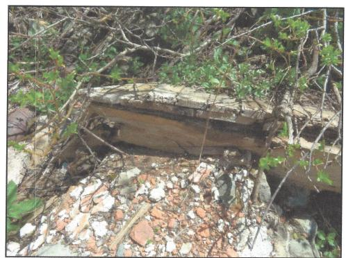
Figure 36. Building floor remnant showing diagonal 1-x-6-in. subfloor topped by 1-x 4-in. tongue and groove flooring set on 3-x-6-in. joist at the Silver Crown Mine (5SA407). View is to the north.
