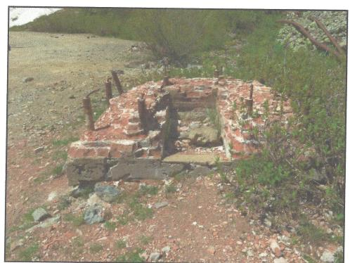
Figure 34. Stone, cement, and brick compressor mount at the Silver Crown Mine (5SA407), looking south-southwest.
