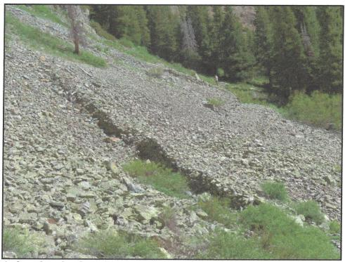
Figure 44. A-shaped avalanche deflector walls looking north-northeast from the southern avalanche deflector wall at the Silver Crown Mine (5SA407).
