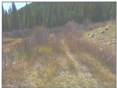
Figure 9. Southern end of the road section within the Bonanza Boy Mill Site, looking southwest. Note willows and grasses growing up through roadbed.
