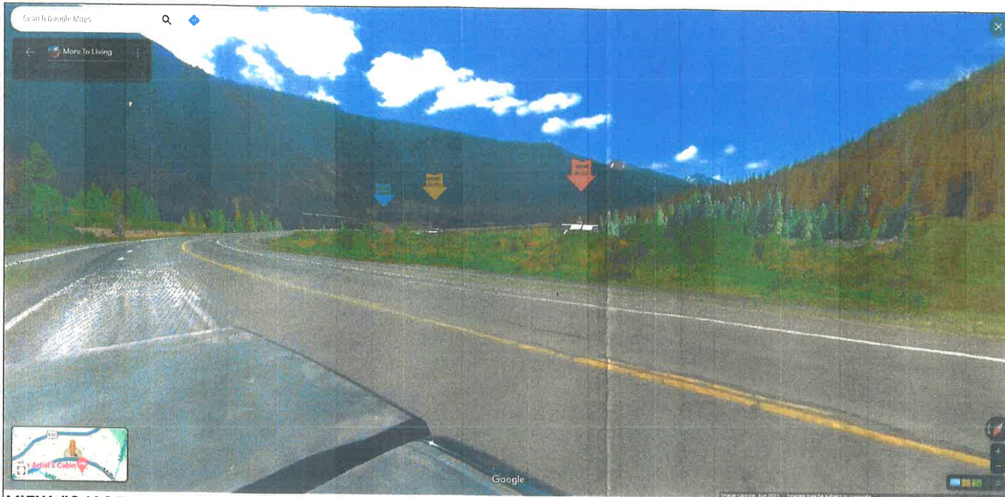
VIEW #2 NORTH-BOUND LANE LOOKING SOUTHEAST ON HWY 550
